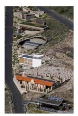
The Development of 25 Bioclimatic Homes is a clear example of the integration of renewable energy sources into building and it shows the different options designed to make use of natural resources to produce electricity: curtain walls and glass roofs with glass-glass photovoltaic panels (made on site) and photovoltaic panels as shadow elements to control solar radiation incidental to the houses.
