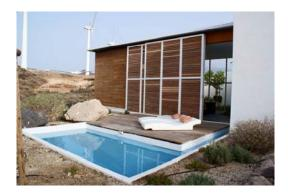
Another notable feature in the Housing Development is a variety of systems used for máximum natural light, which mean that it enters directly into the home's interior spaces (Core system) or areas adjacent to the house's exterior (Perimeter system). The use of raised windows, sunshades, skylights and side lighting also reduce power costs.
